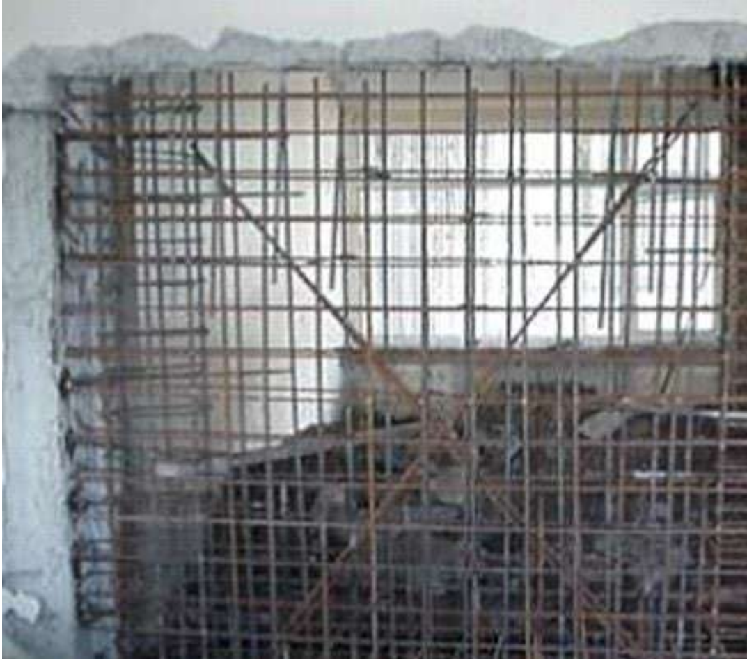
Fig 2: Additional Shear Wall
