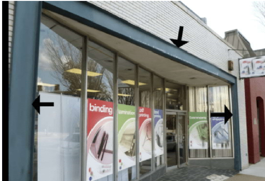
Large building entryway moment frame
