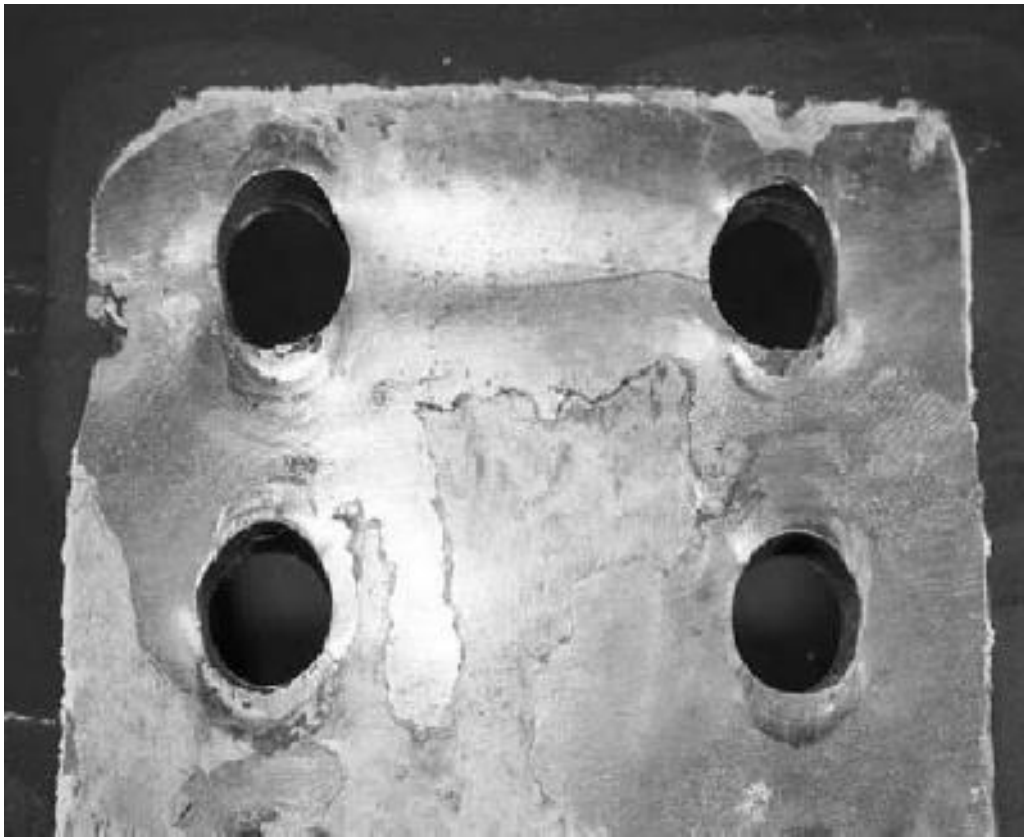
Figure 10.16 Bearing failure of plates
