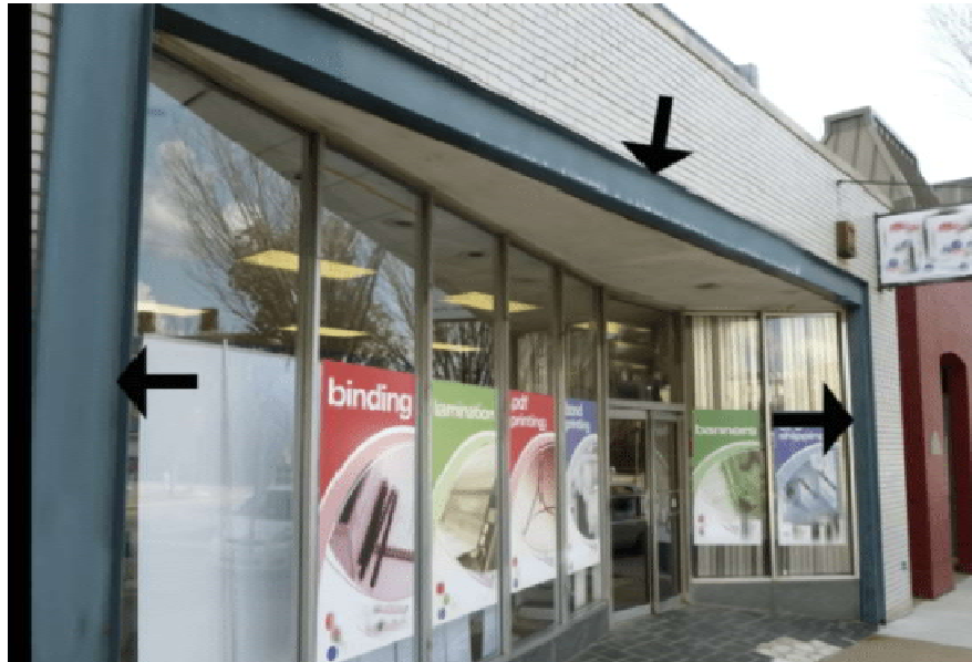
Large building entryway moment frame
