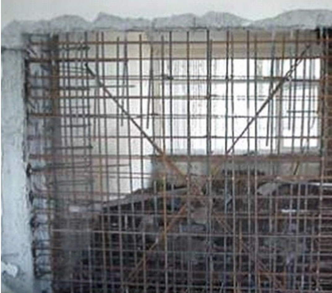
Fig 2: Additional Shear Wall
